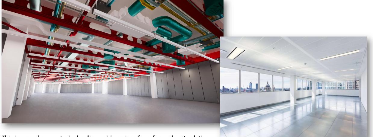
This image shows a typical ceiling void services for a fan coil unit solution.
